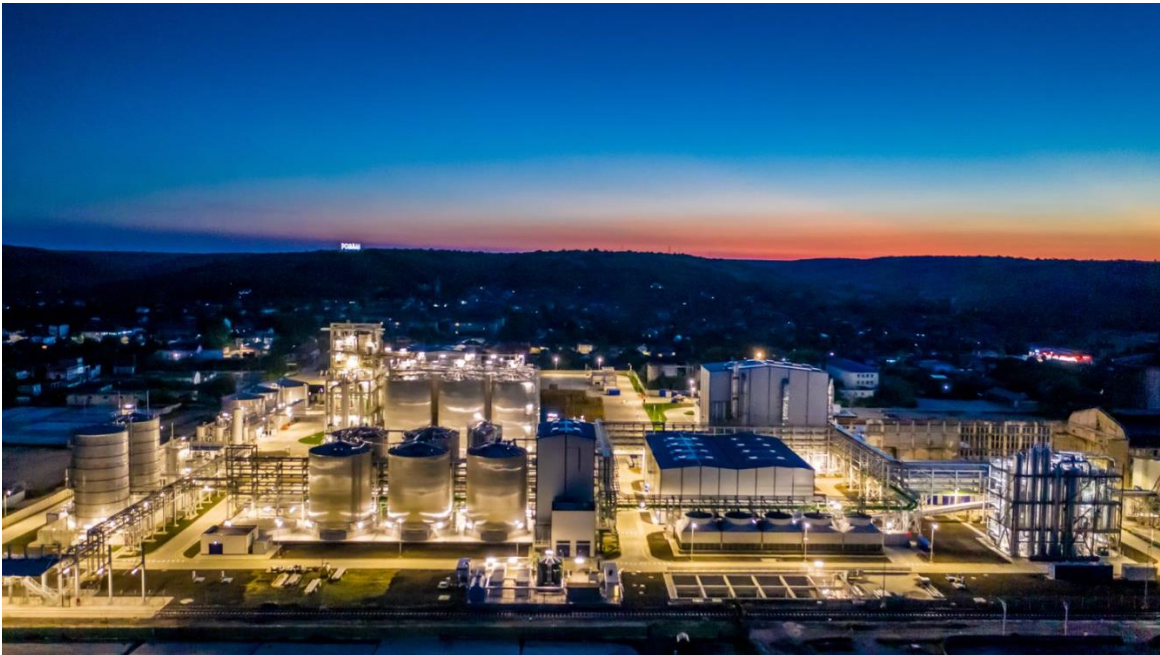
Clariant's flagship sunliquid® cellulosic ethanol plant in Podari, Romania. (Photo: Clariant)
